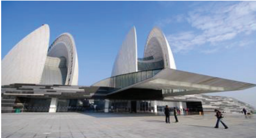
Figure 2 – Exterior Zhuhai Opera House
