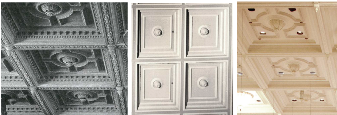
Fig. 8. Ornamentation of ceiling, Left: original; middle: 1962, right: after renovation 1998 (9)
